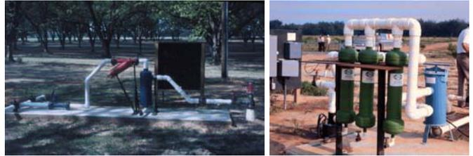
**Figure 19.** Screen filter and vortex sand separator installations.
