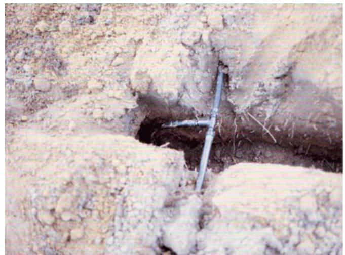
**Figure 16.** Connecting lateral line to PVC.
