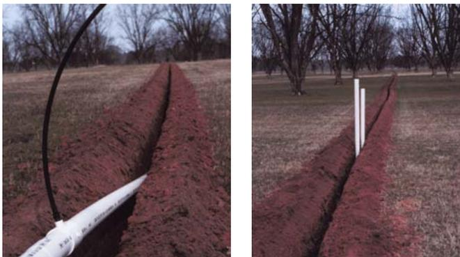
**Figure 4.** Installing PVC mainline.
