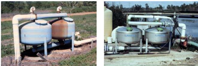
**Figure 18.** Sand (media) filter installation.
